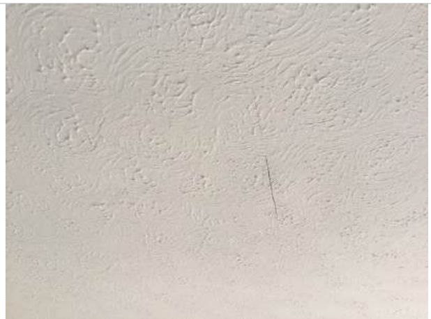
22. Cosmetic ceiling crack in bedroom 1
