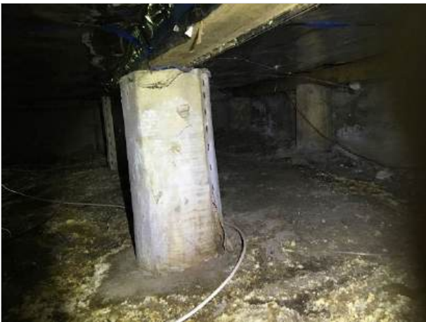
9. Typical pile and subfloor moisture barrier
