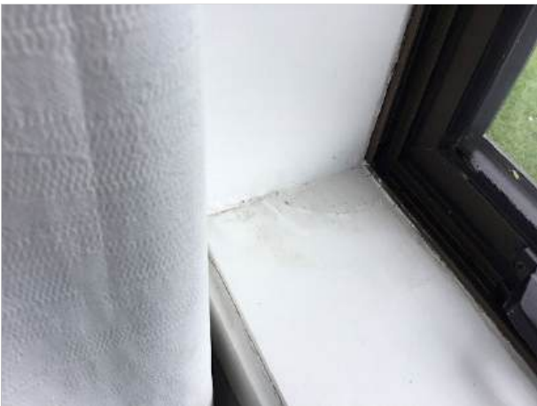
21. An example of unfinished reveal repairs
