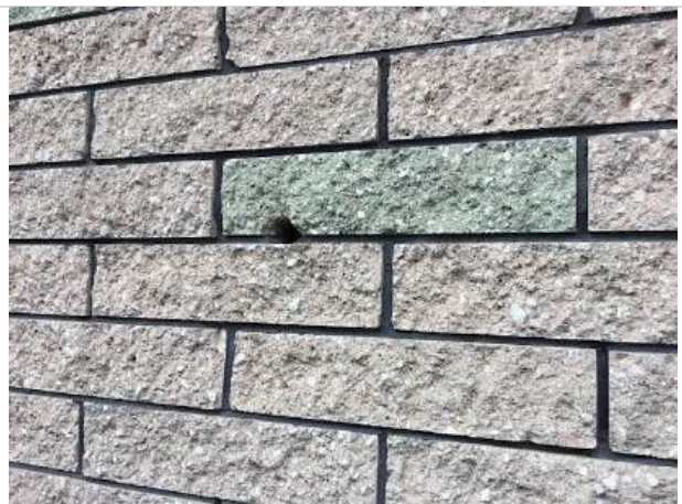
24. Hole from old toilet overflow pipe should be sealed
