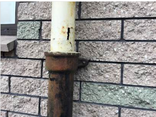
23. Sewer vent pipe corroded
