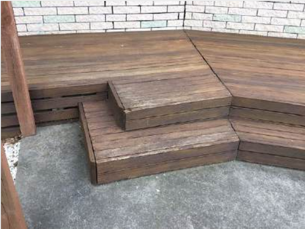
25. Deck due for recoating
