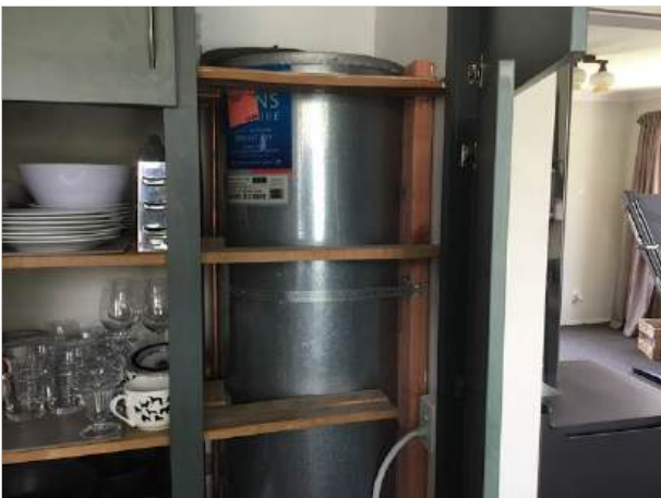
11. 180L mains pressure HWC manufactured 2011
